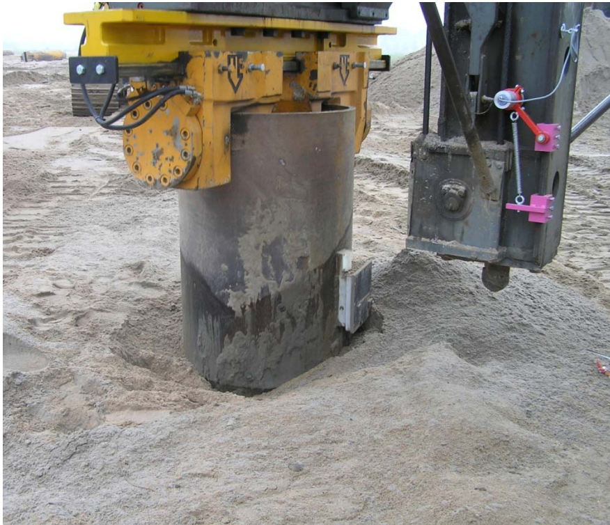
on pile head mounted unit by final depth
