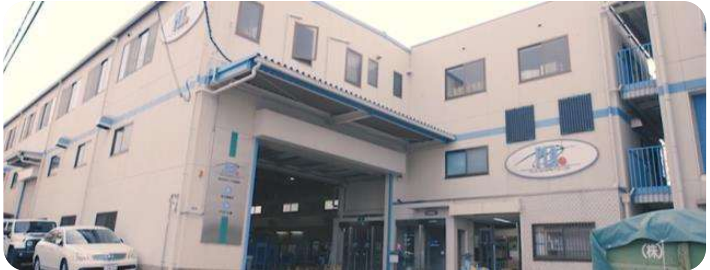
Main Office and Factory (Suita-city, Osaka)
