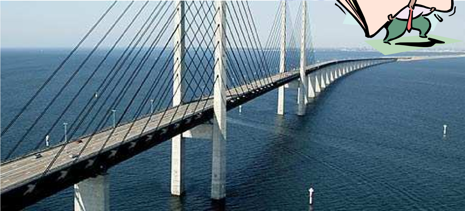
... use tools to build a bridge
